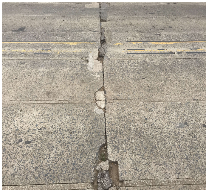
PHOTO 1 Description Typical spalling over the intermediate bents.
