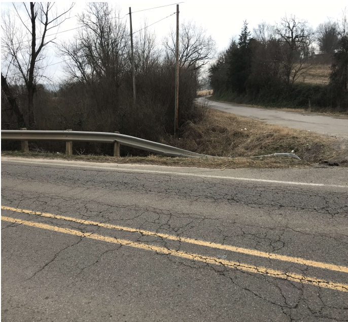
PHOTO 1 Description Southwest approach guardrail damage.
