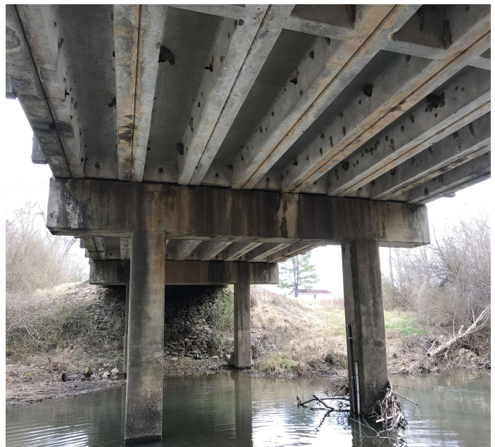
PHOTO 2 Description Bent # 3 cap spalling.
